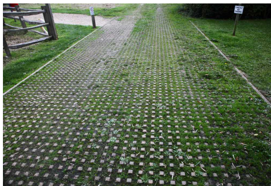
Sympathetic use of grass pavers to achieve the existing farm access
